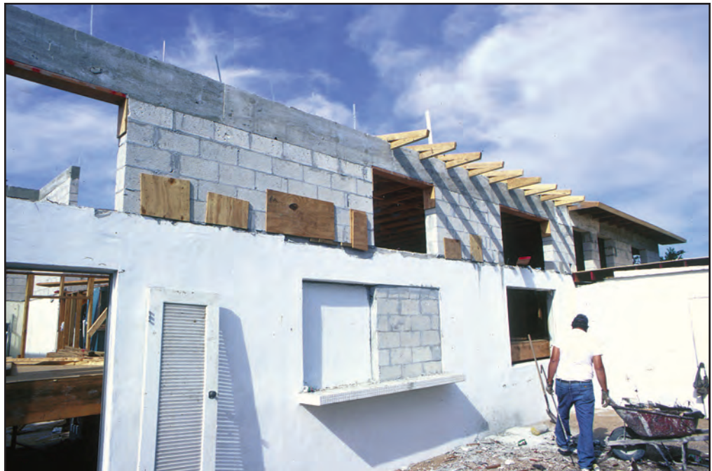
Figure 67 The extended first-story walls.
